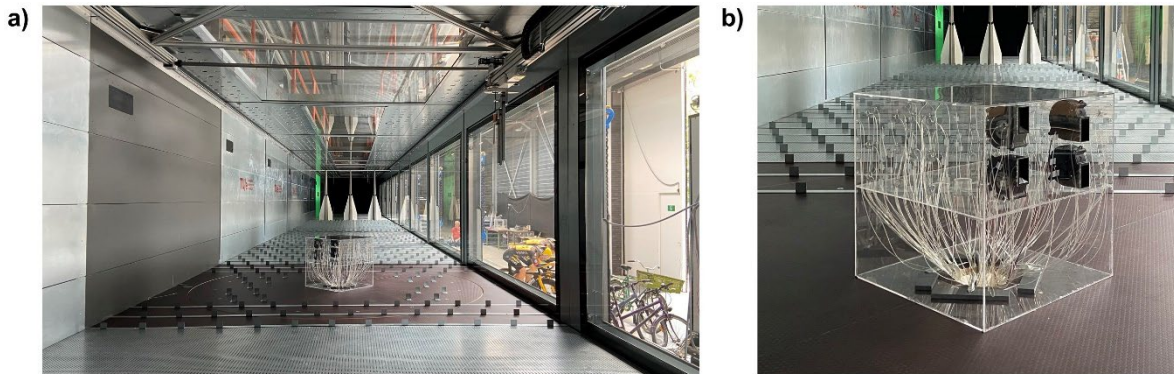
Figure 1. a) Photograph of the building in the wind tunnel; and b) close-up view of the building with mechanical ventilation system.
